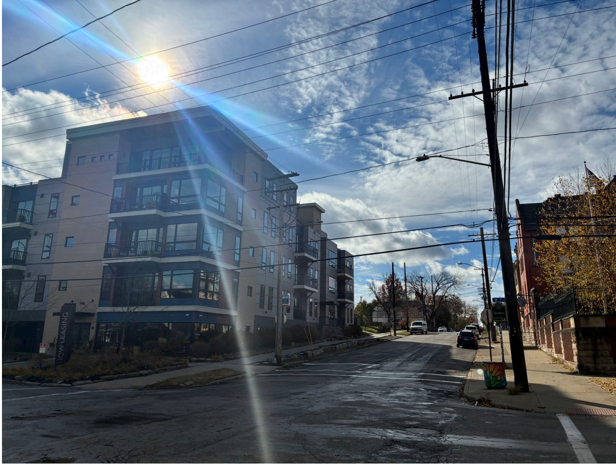
W 7 th St & Jefferson Ave, looking southwest
